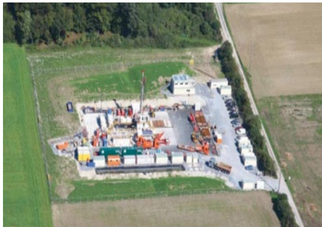
Fig. 1: Drilling site with drilling rig and auxiliary installations (Schneble et al. 2011).
